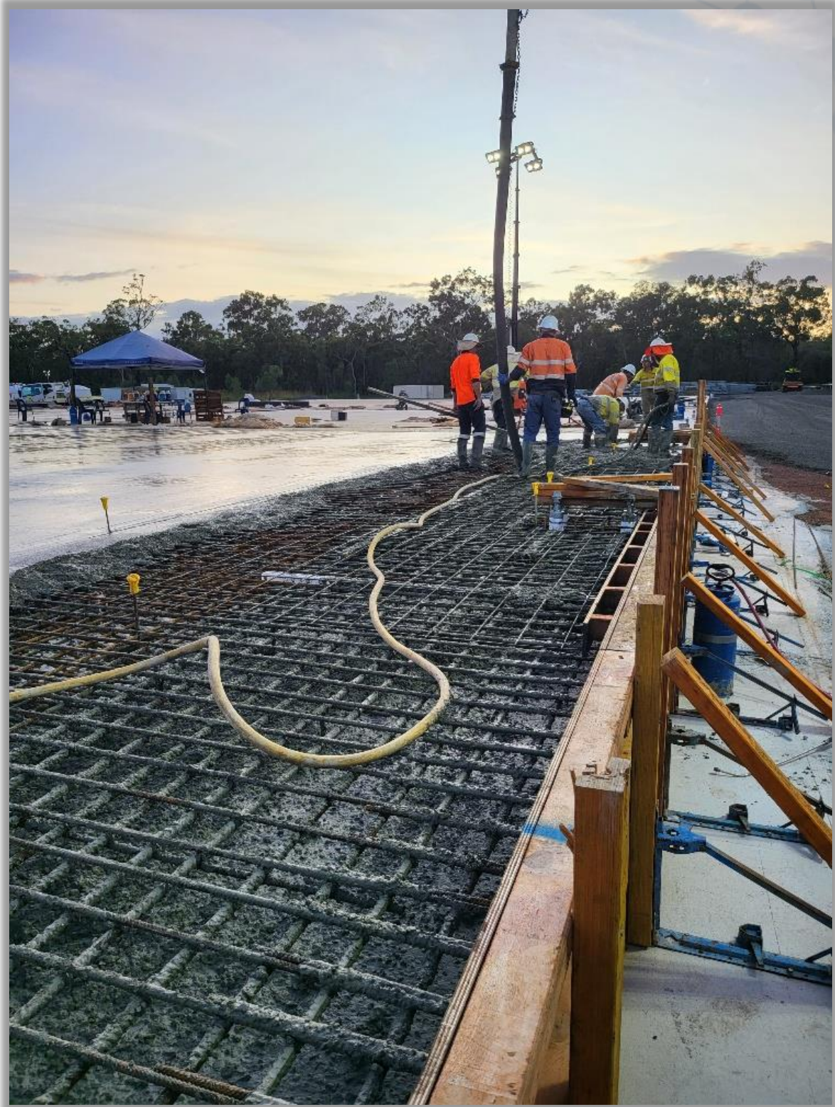
Pouring the eighth and final main PPF building slab
