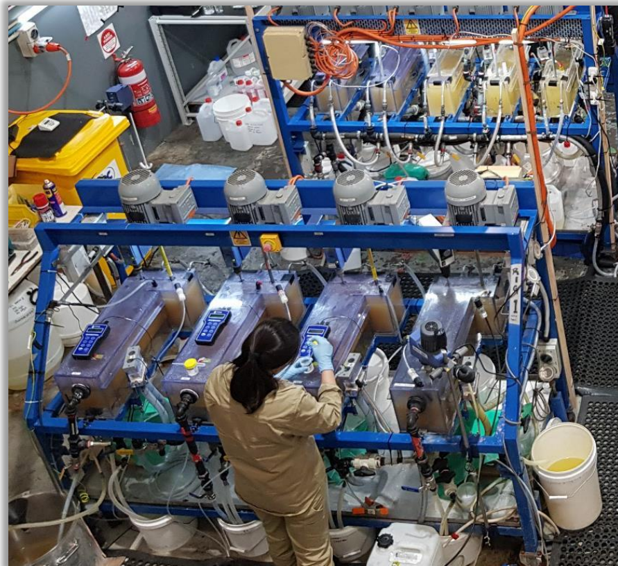
Pilot Plant – Solvent Extraction Circuit
