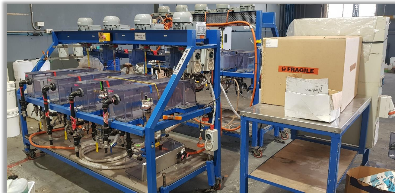
Figure 2: Solvent Extraction cells for the pilot plant installed
